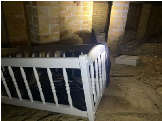
Example of timber on the ground in the subfloor
