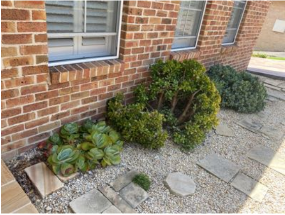
Example of vegetation located close to the building
